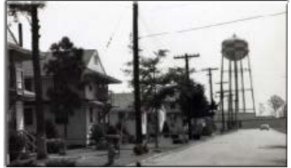
Water tower on base
